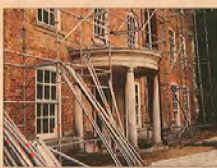
Restoration work under way at Rivenhall Place in Essex, England.
